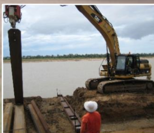
EXCAVATOR MOUNTED PILING EQUIPMENT
